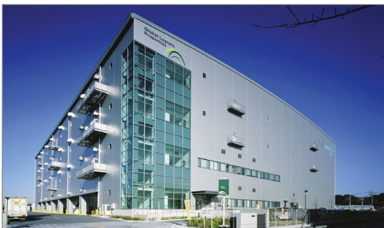
Global Logistic Properties building, Brazil
