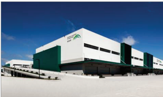
Global Logistic Properties building, Japan
